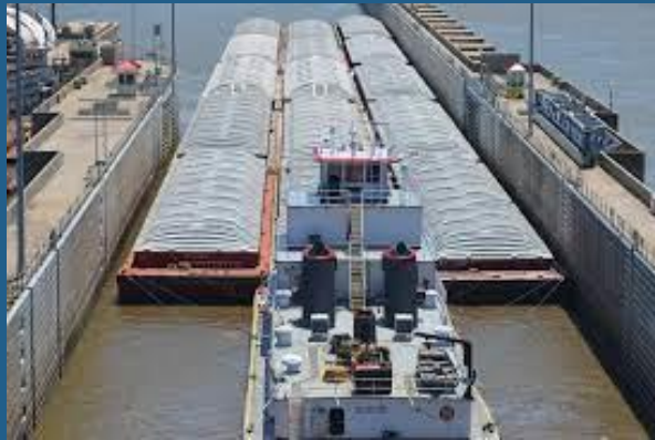
Boat and barges in river lock
